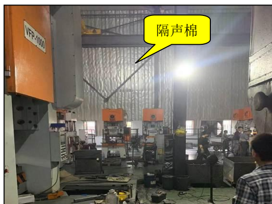
车间墙壁加装隔声棉
